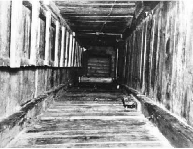
One of the tunnel shafts, well shored with bed boards. Just over 2 feet in length, these dictated the dimensions of Tom, Dick and Harry.
