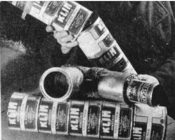
"Klim" milk powder was sent in our Red Cross parcels. The empty tins were joined together to form pipes, used for the tunnel ventilation and as a temporary flue for the stove when it was removed from the tunnel entrance.
